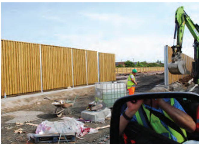
Location 7: New Road looking E – Railway to left
