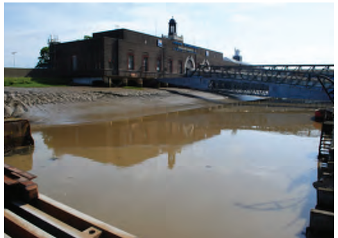
Location 1: Looking NE. Cruise Terminal from Operational end of Landing Stage
