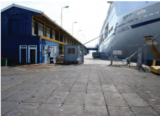
Location 1: Looking E along passenger Landing Stage
