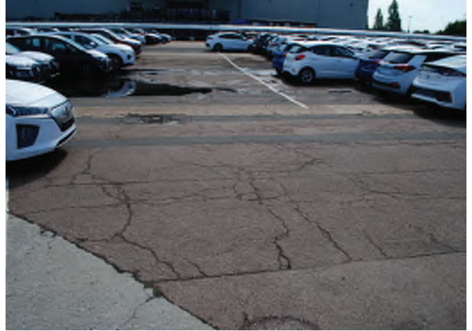
Location 11: Former rail lines visible in repaired tarmac
