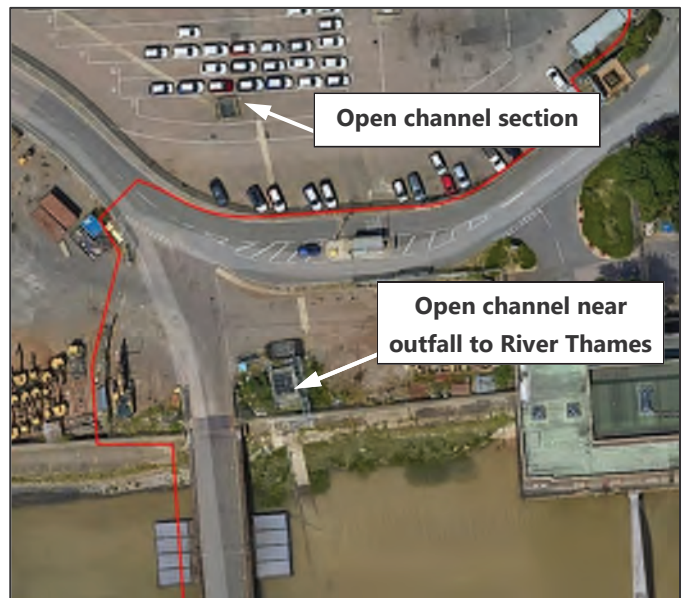
Figure 3-1 – Open channel sections of otherwise culverted watercourse (on- / adjacent to western boundary).
