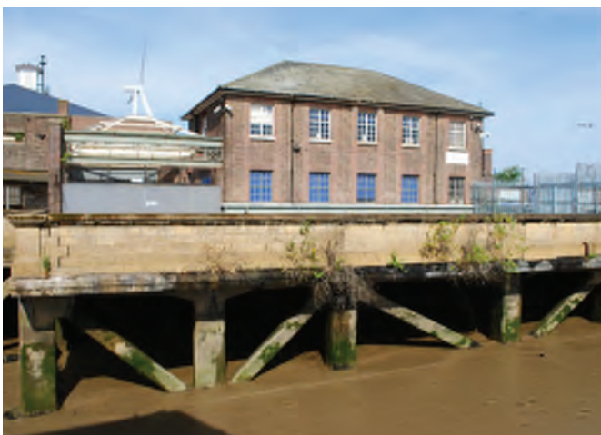
Location 3: Looking W at Cultural Centre (E end of Rail Station building)
