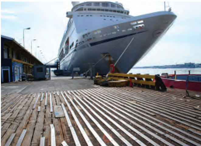
Location 1: Looking E along passenger Landing Stage
