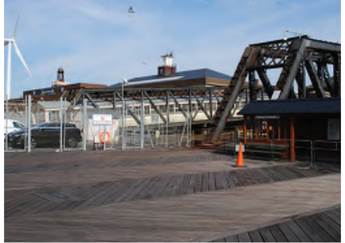
Location 2: Ferry Terminal
