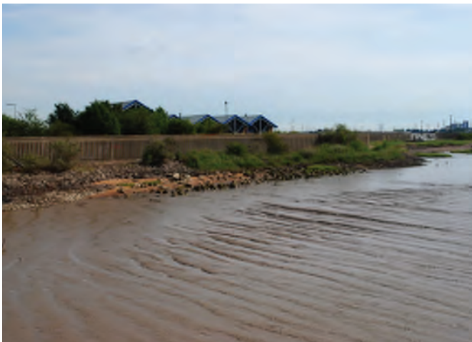
Location 3: Looking NE towards River Wall
